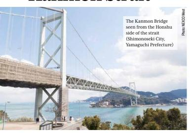
The Kanmon Bridge, which connects Japan's main island of Honshu and Kyushu, the large southerly island, is a 1,068-meter-long suspension bridge built using an innovative construction method. It represents a milestone in the history of suspension bridges in Japan.
